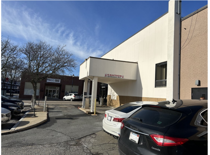
Former Bank Drive-thru
